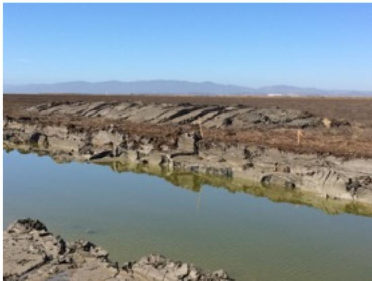
Figure 8. 22 marsh mounds have been built from the soil material excavated from the channel. Marsh mounds will offer high tide refuge for marsh wildlife adjacent to the channel alignment.
