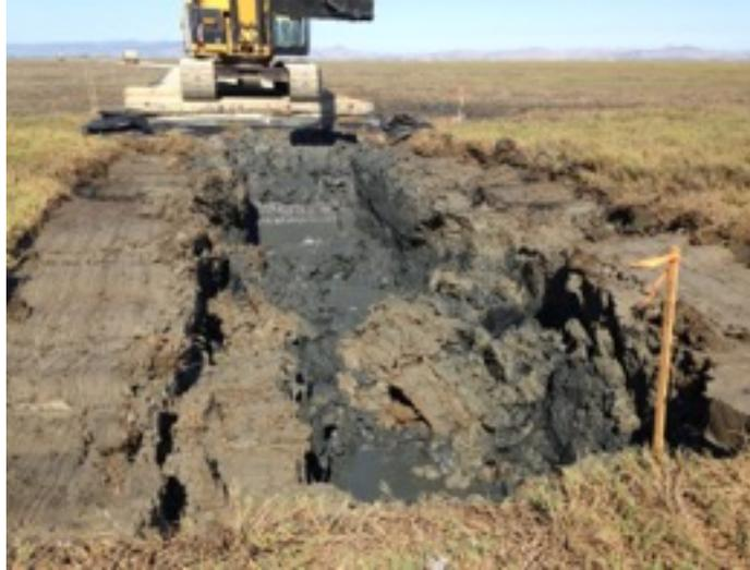
Figure 7. Hanford excavated the southern end of the main channel alignment with an approximately 16ft top width and 5ft depth. The channel top width gradually widens as the channel nears Sonoma Creek to 50 ft top width and 7.5ft depth from marsh elevation. Because of difficult construction conditions and substrate consistency, the side slopes were modified from a 1:1 to a 3:1 slope ratio to ensure channel banks do not slump more than expected.
