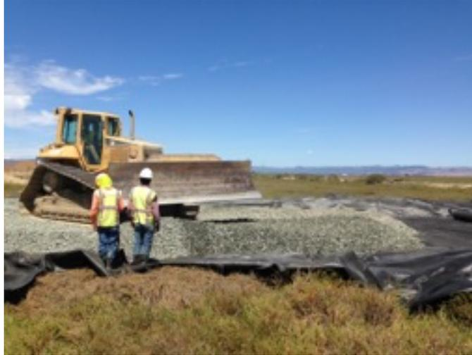
Figure 5. Hanford designed and constructed a 18"-24" thick, permeable access road from adjacent farmland levee to the center of the marsh and Sonoma Creek Enhancement Project Area. All road material was removed simultaneously with Hanford's excavation of the main channel.
