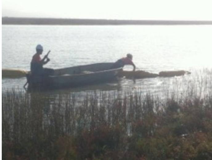
Figure 9. An exclusion curtain was placed to inhibit the access of marine wildlife such as fish and mammals into the construction zone and stop suspended sediment from entering Sonoma Creek and San Francisco Bay.
